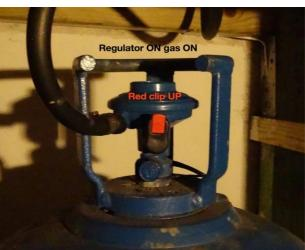
To connect the regulator; place it on the gas cylinder, lift the red clip, and turn the black knob clockwise. When the red clip points upwards, the regulator is connected and the gas is on.
